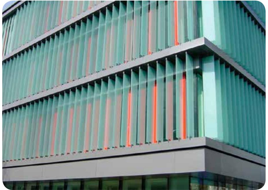
Simple, effective shading systems are key to a successful passive design.
